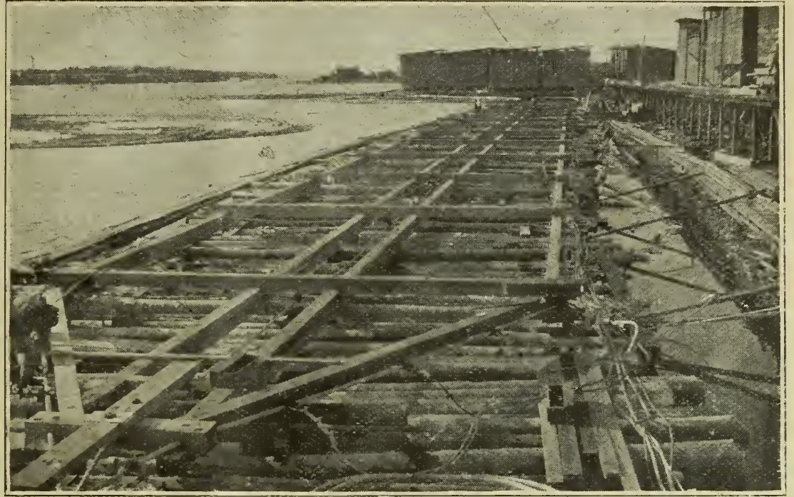
Fig. 1.—Base of Float in course of construction.
